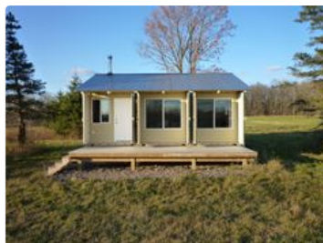
The Tin Can Cabin was built from 3 shipping containers
