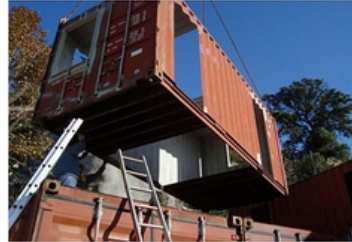
Plans in Motion: Shipping Container Home-Building Photos
