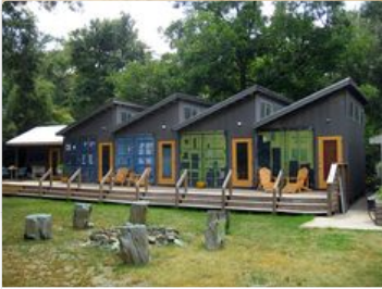
studios built with shipping containers
